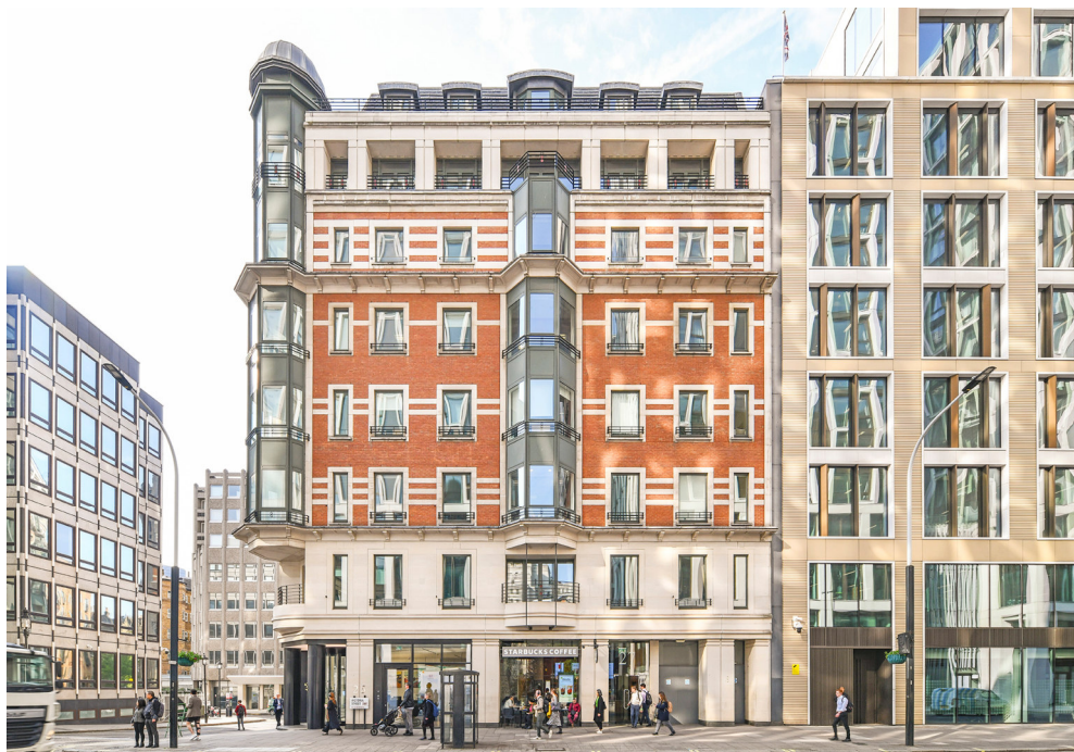
25 Victoria Street, Londen © Delancey Real Estate
